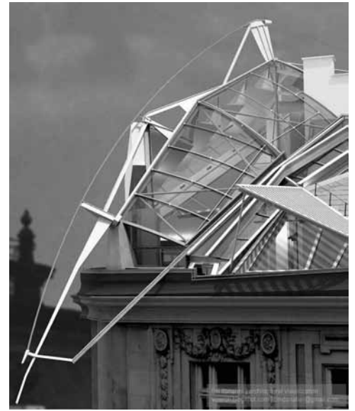
Coop Himmelblau, Vienna Office Chord, 1990
