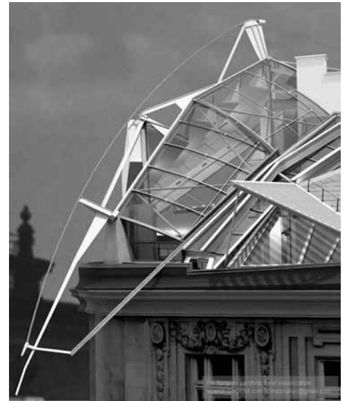
Coop Himmelblau, Vienna Office Chord, 1990
